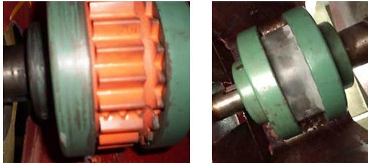
Figure 2 The Most Commonly Found Elastomeric Couplings- Not Listed/Approved for Fire Pump Systems (picture on right shown with coupling boot)
