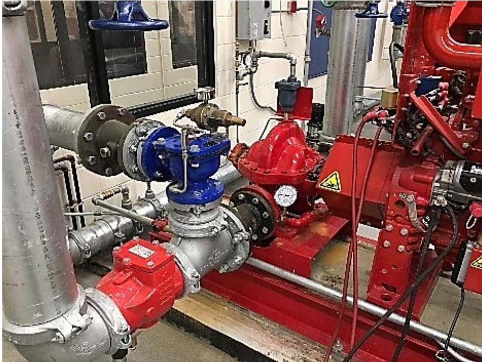
Figure 1 Centrifugal Fire Pump Assembly
