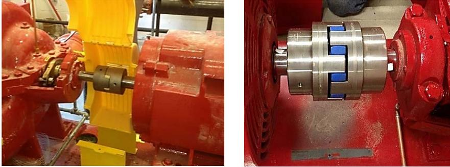
Figure 4 The Most Commonly Found Jaw Couplings (with elastomeric component) Listed/Approved for Fire Pump Systems
